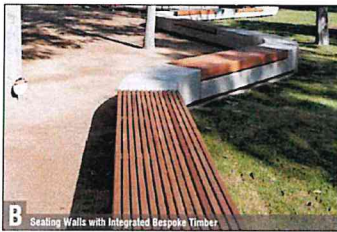
B Seating Walls with Integrated Bespoke Timber
