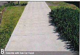
B Concrete with Saw Cut Finish
